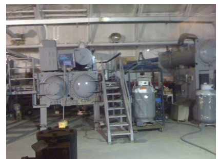
Chena Resort Geothermal Generator
