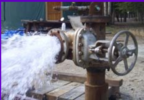
Geothermal Wells Provide Hot Water (~165F)
